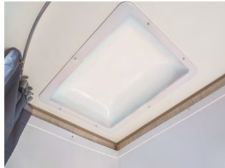
Skylight over Shower
